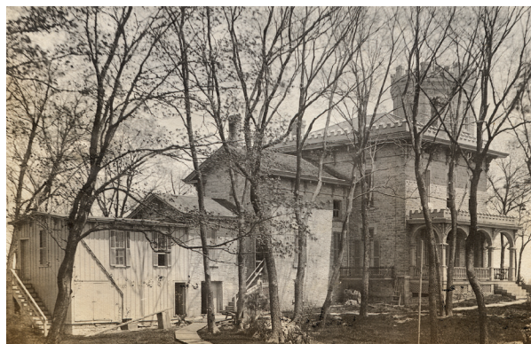
This view from the southwest was taken in 1901, but the house looks much the same today.
