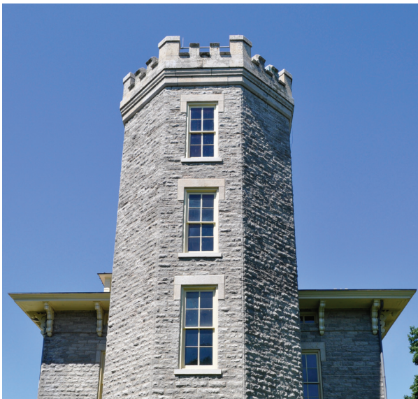
The Gothic style tower is topped with crenellations, and distinctive hood moldings outline the castle windows.
