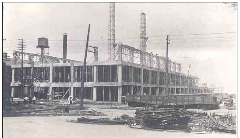
The East wall of the third floor is taking shape in this late 1917 view.
