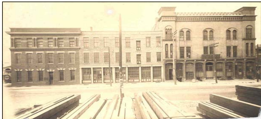
West Water Street building formerly known as "Norman Hall"
